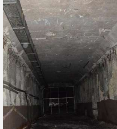
The concrete volume
