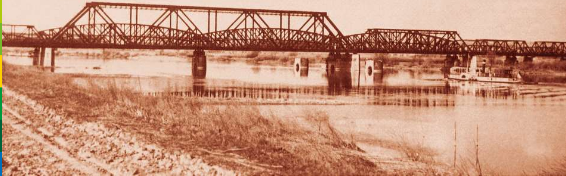
Two bridges (railway and road) 1930 – 1945
