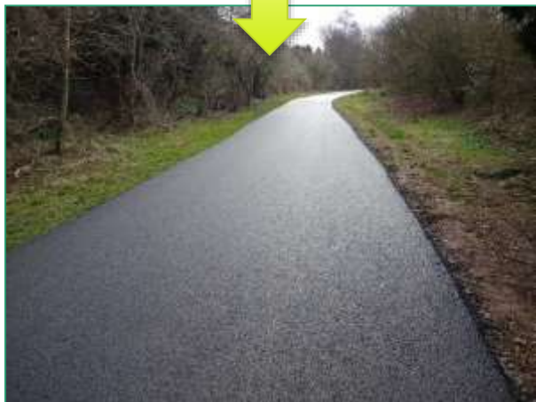
PATH WIDENING 3m to 4m
